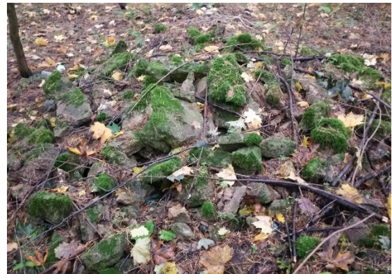
Figure 27. Likely remnants of a stone wall (though possibly an ohel) at Trzcianne. The rubble will need to be removed and a fence or other boundary marker installed.
