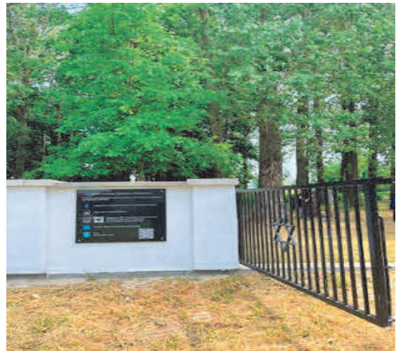
Figure 29. Markuszów Jewish Cemetery - new fence and wall around part of the cemetery; the remainder will be delimited with a plant hedge.
